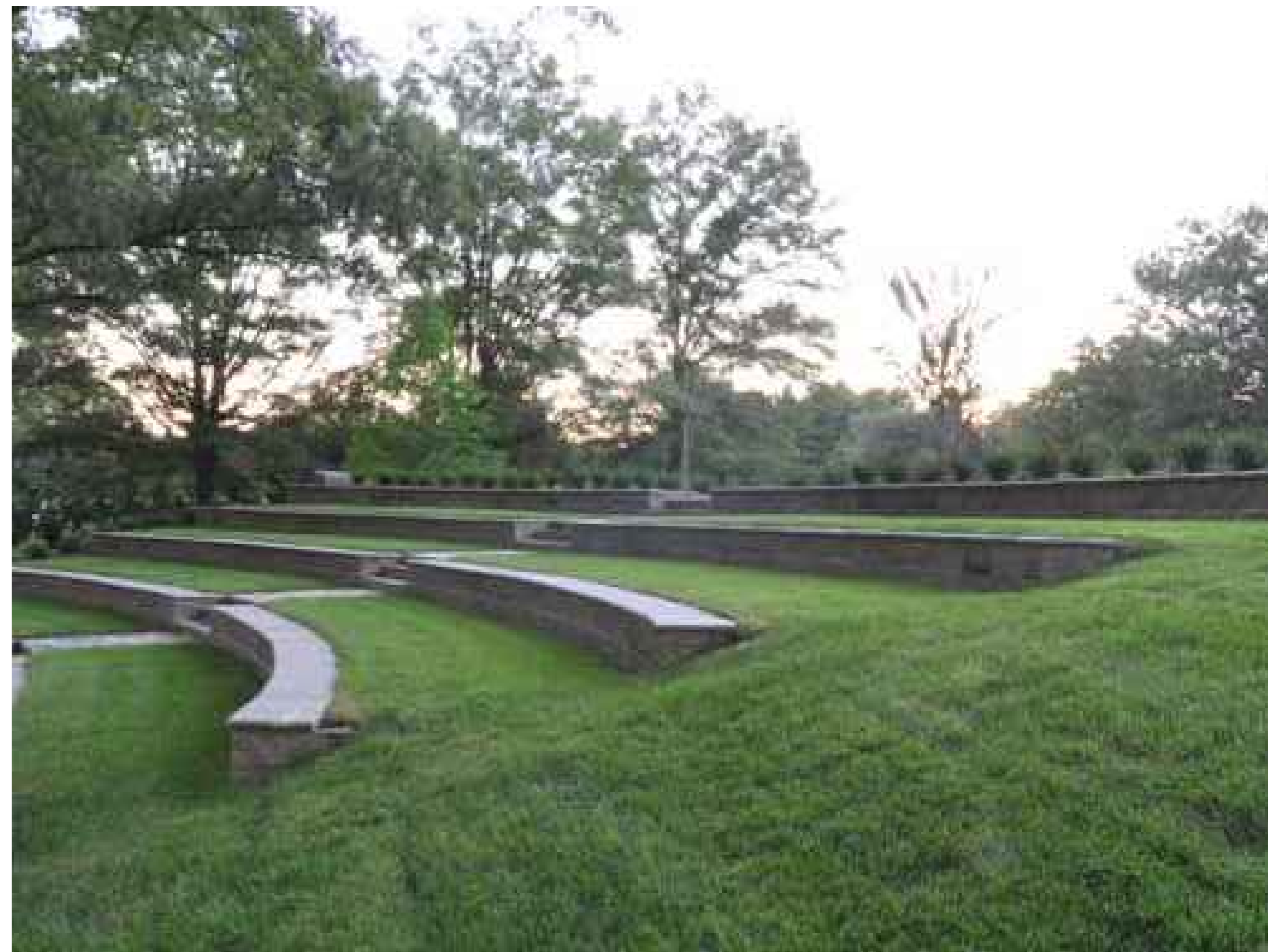
C.I.P. CONCRETE SEAT WALL
